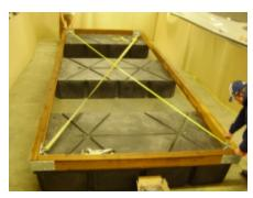
If frame is out of square a long strap can be used to pull it square. Once frame is square secure it by tightening the bolts.
