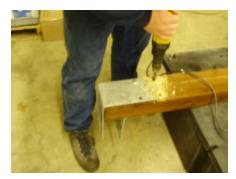
Drill and install remainder of carriage bolts, as shown.
