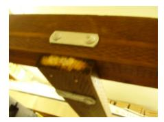
Note that the carriage bolts are installed so that the flat head is out and on the bottom side. It is safer to have the bolts installed this way to prevent possible head injuries to a person should they swim under the dock.
